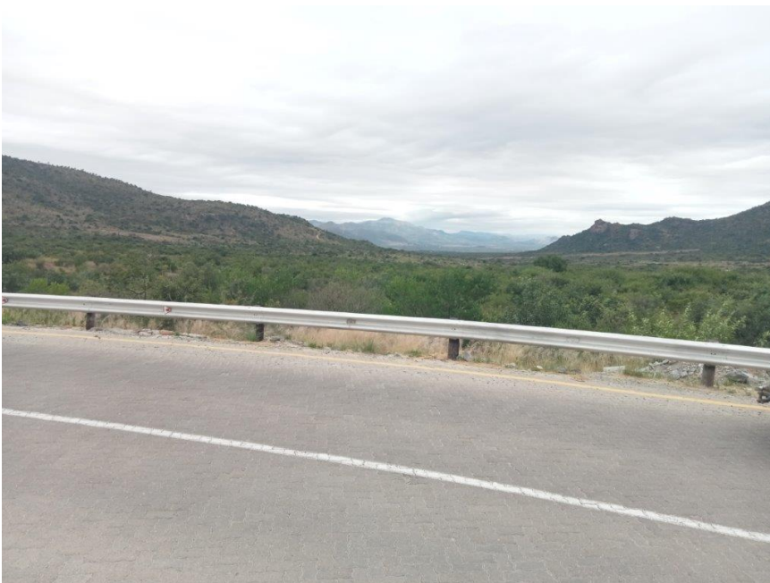
Figure 10: View of where the planned mining road will wear off the existing tar road.
