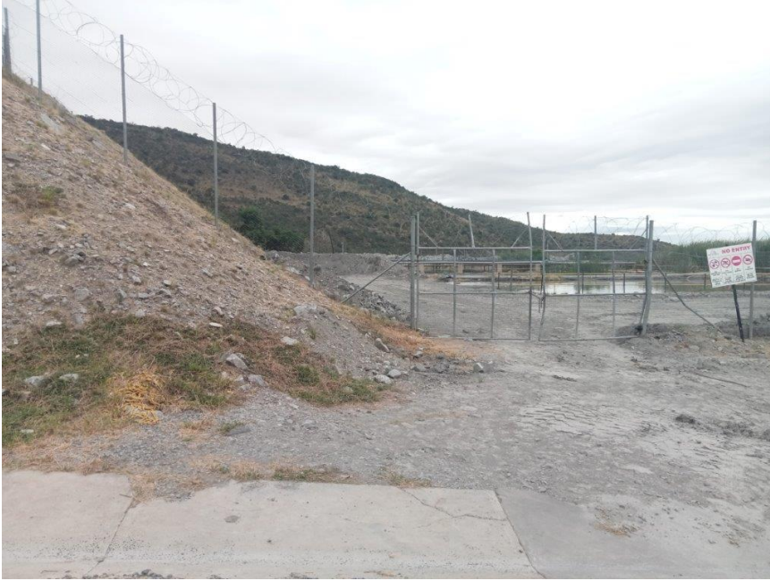
Figure 9: Start of the planned road at the existing plant area.
